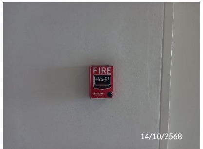
Fire Alarm Manual Station
