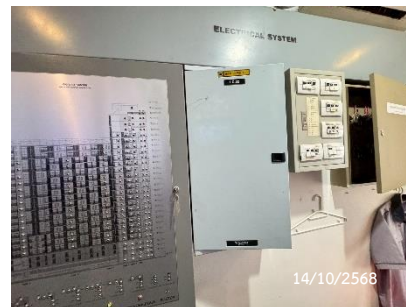
Graphic Annunciator Fire Alarm System
