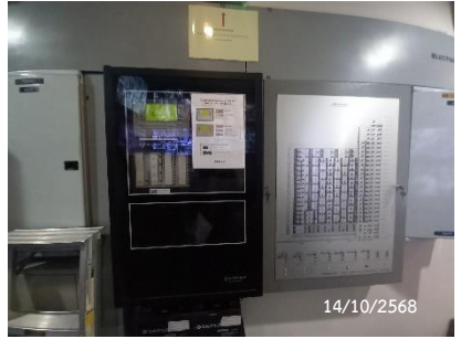
Fire Alarm Control Panel
